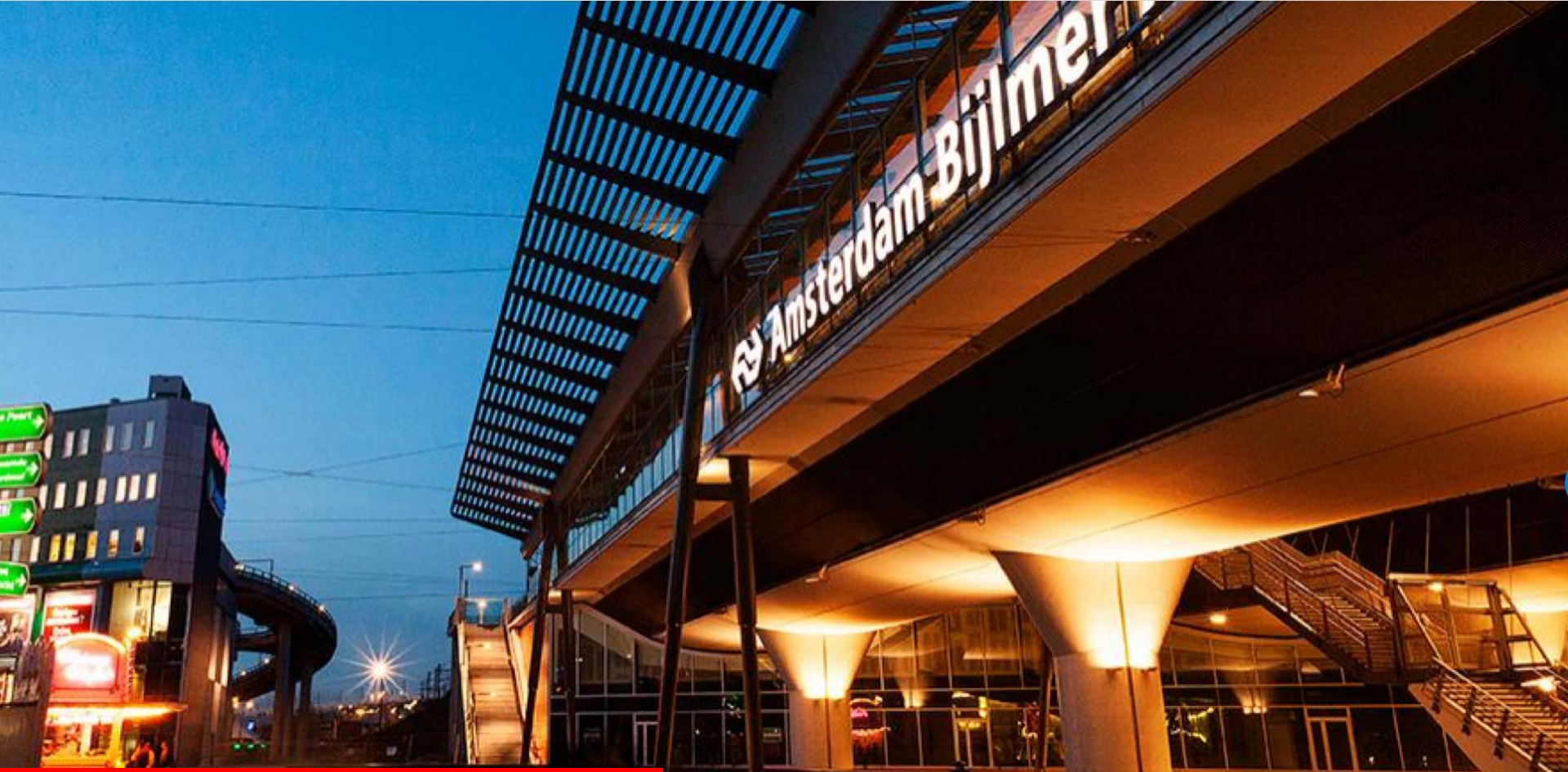
Station Bijmer ArenA
